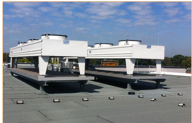
The Water Resources Act (WHG) and the Plant Ordinance (AwSV) regulate the handling of substances hazardous to water. The glycol protector made of stainless steel or aluminum AlMg<sup>3</sup> helps to meet this legal requirement.
